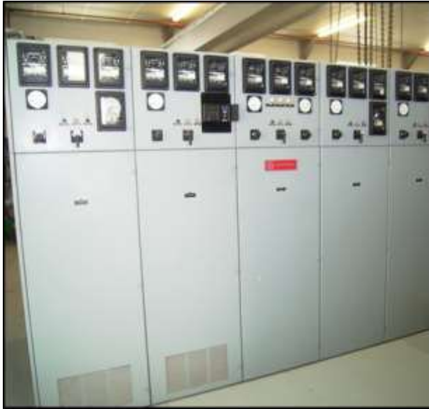
The existing switchgear is shown above. New medium-voltage switchgear installed in a main-tie-main configuration will replace the existing switchgear to improve reliability and redundancy in the electrical system.
