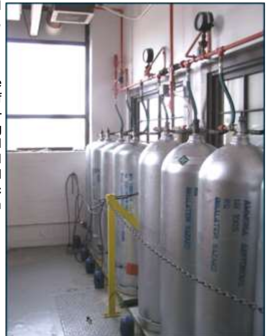
The existing anhydrous ammonia storage facilities are shown in the photograph. A new liquid ammonium sulfate storage and feed system will eliminate safety concerns associated with storing and handling compressed anhydrous ammonia.
