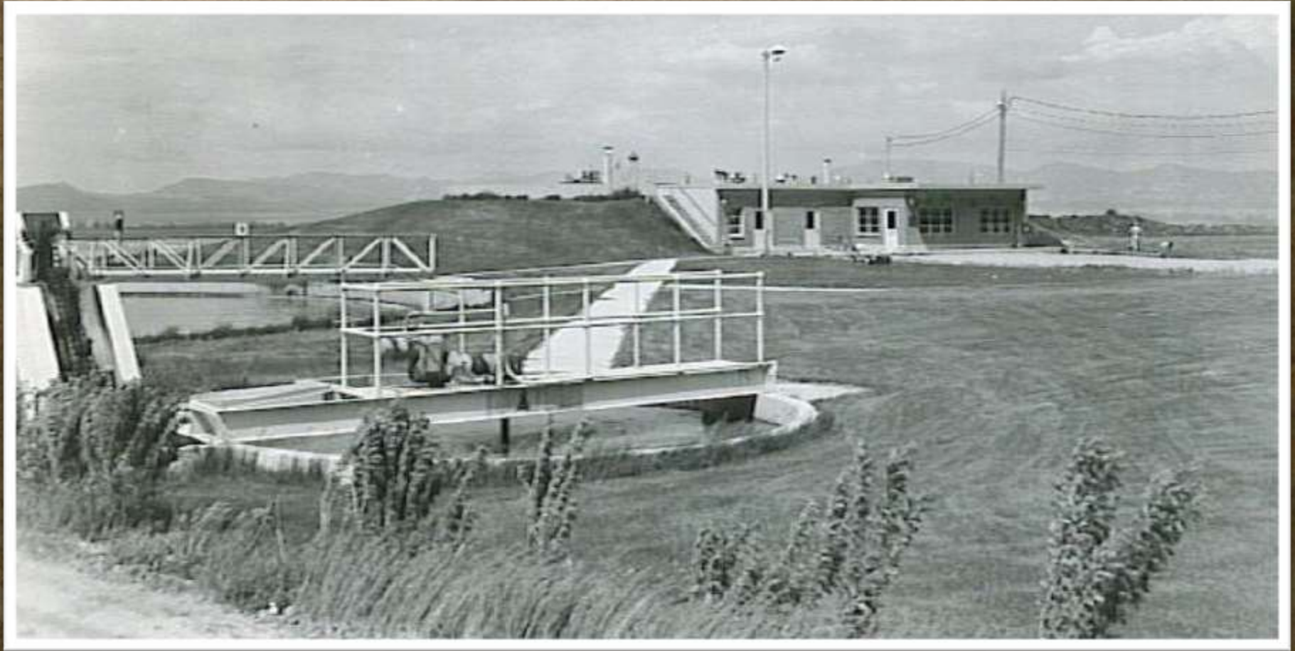
Grit Chamber and Primary Clarifier - ca 1960s
