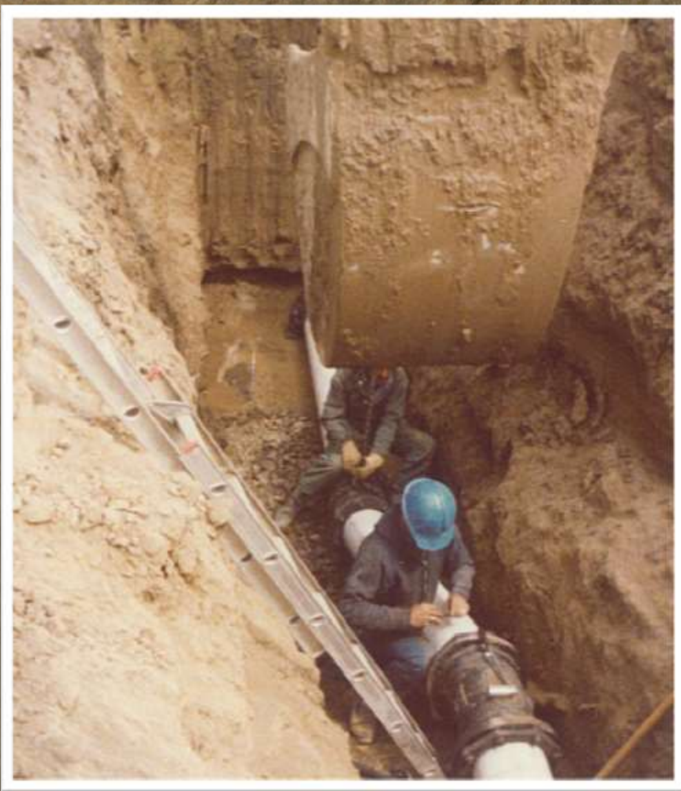
Installing Pipe (60s or 70s)
