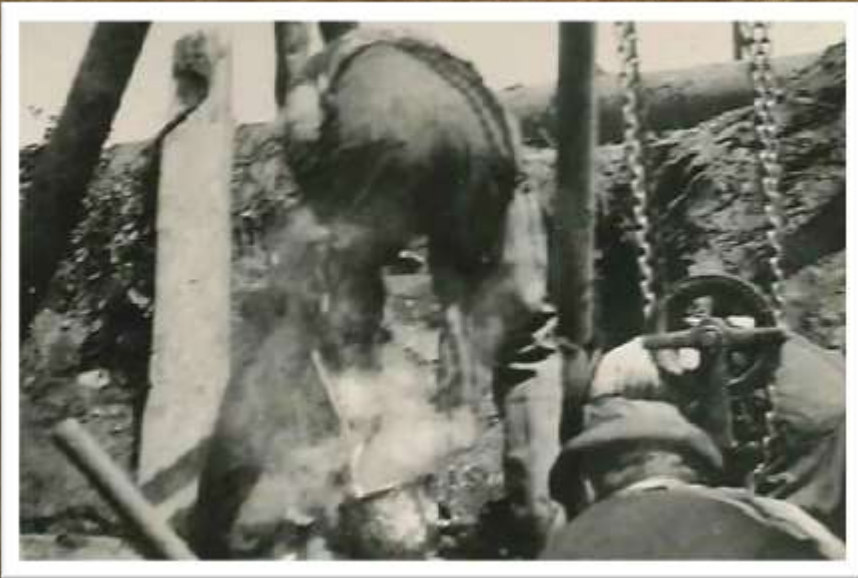
Bert Lay Pouring a Lead Joint
