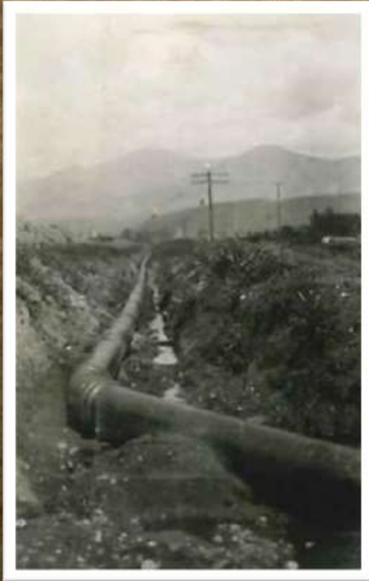
Cast Bend 100 ft. N. of Valve House
