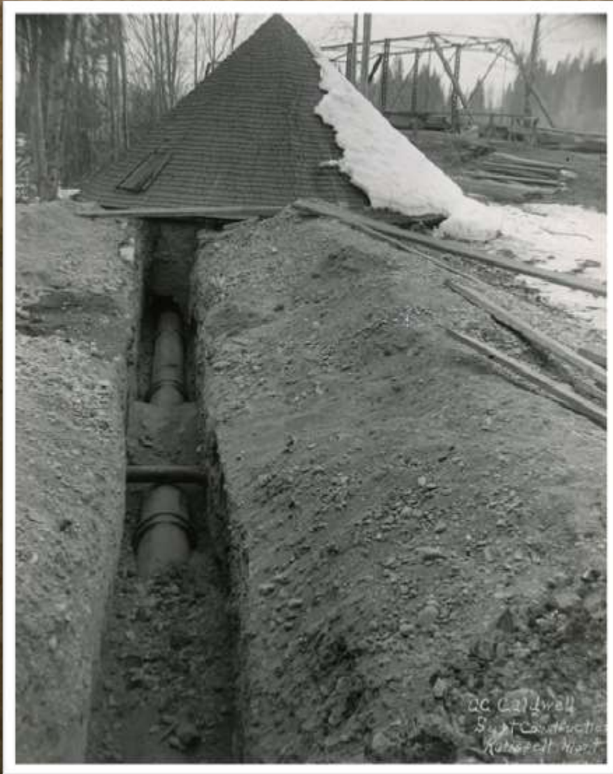
Water Works Suction Lines from Well to New Pump
