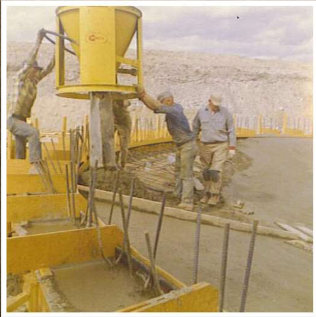
Pouring Secondary Clarifier Floor- ca 1980
