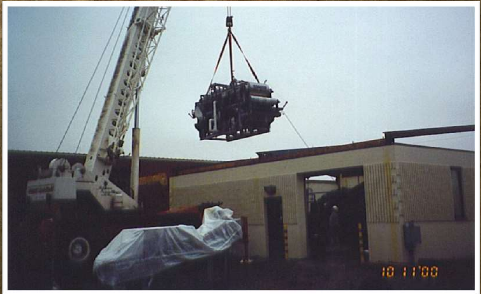
Installing Second Belt Filter Press, 2000
