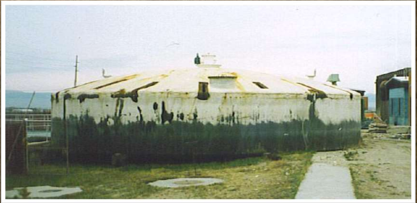
Digester Floating Cover Removed
